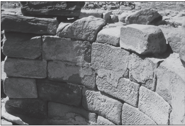
5. Room R wall with quarried Nabataean dressed blocks and extant wall plaster. (WRRP).
