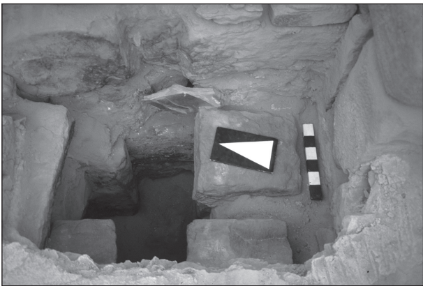
6. Room W hypocaust with stone pilae, stone pilae-covering slabs, flue vent, and plaster layers of hanging floor. (WRRP).
