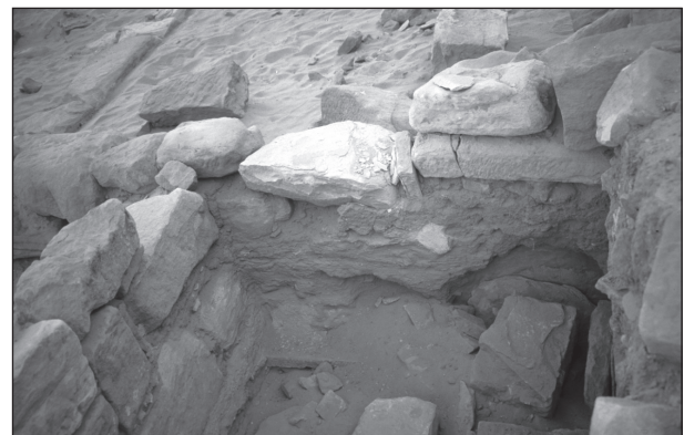
14. Room L vandalism: removal of floor stones and digging into the missing lower section of the wall between Rooms L and K. (WRRP).
