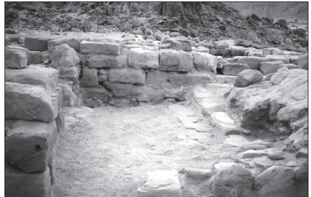
15. Room M after cleaning in 1996 revealed the edge of the frigidarium ’s basin. (WRRP).
