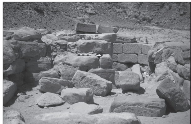
4. Room Q and corridor to Room R filled with tumbled blocks prior to the WRRP's 1996 cleaning. (WRRP).
